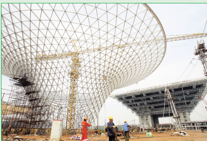
One of the six "Sunny Valley" horn structures on the Expo Boulevard which leads to the China Pavilion (far right). The horns are designed to collect rain water and disperse sunlight to the underground levels of the three-story boulevard.
